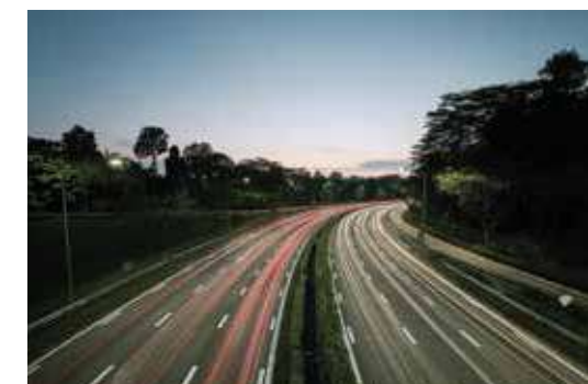
Future North-South Corridor
